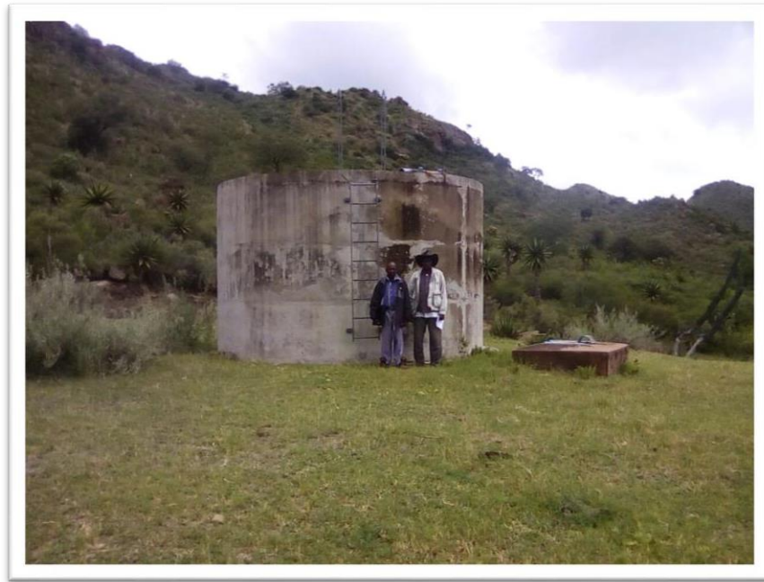
Figure 19: Reservoir at Maroga/Phalatseng (seen here is Nduna’s subjects)
