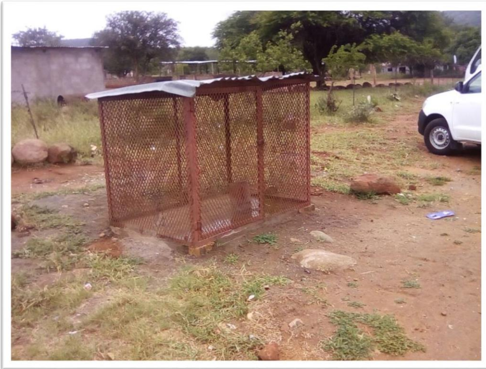
Figure 17: Fenced Borehole at Kampeng Section
