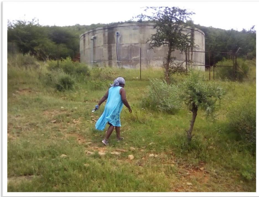
Figure 14: Reservoir at Kampeng Section
